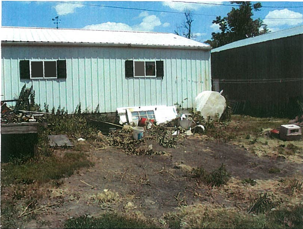
Date: 06/06/2012 Time: 1204 Direction: N Photo by: M. Weber Exposure #: 7 Comments: Former location of a camper and assorted liquid propane cylinders.
